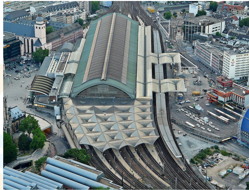
Köln Main Station
